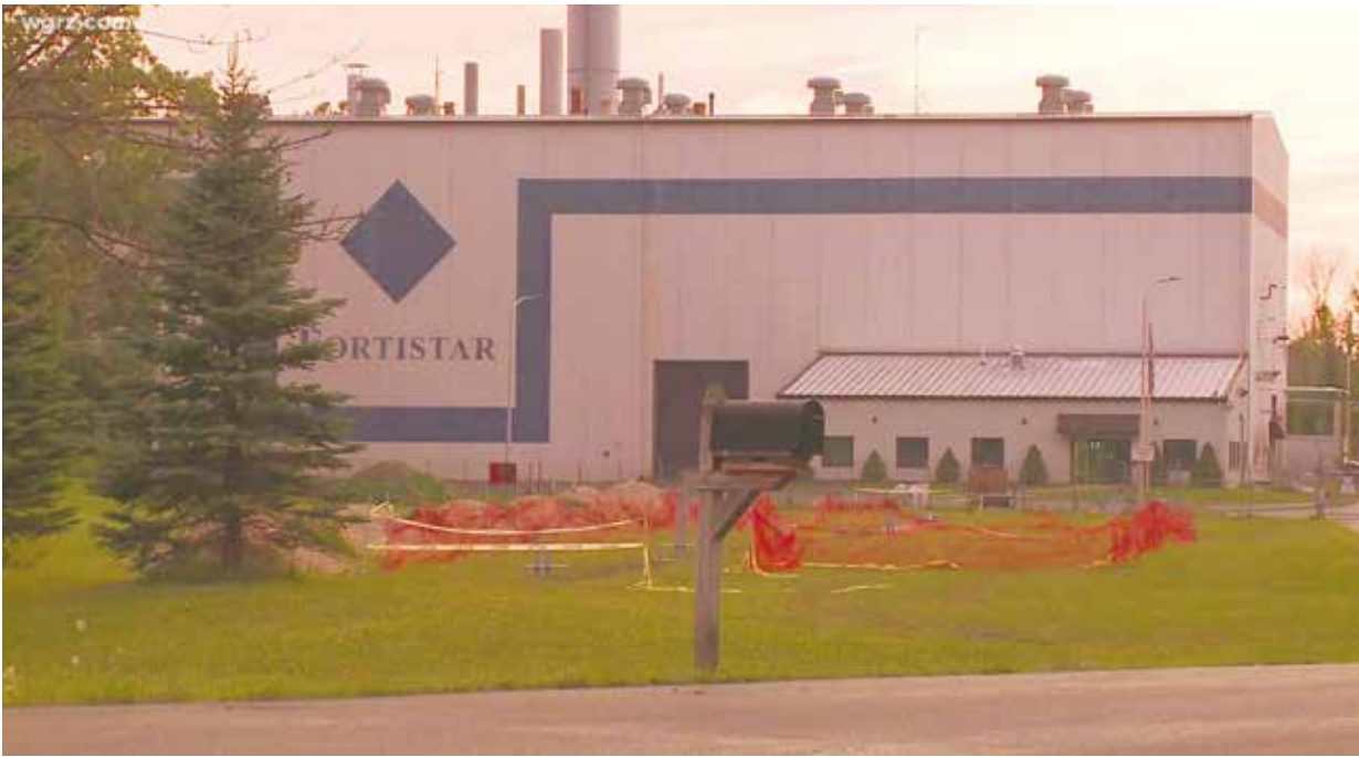
Fortistar gas plant in North Tonawanda, New York
