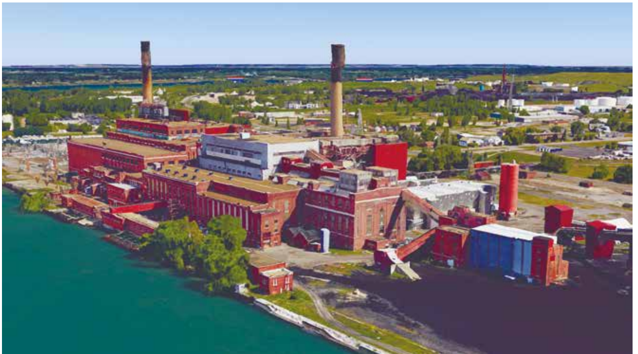
Huntley Coal Power Plant, Tonawanda, New York
