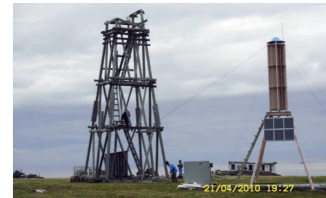
Cape Chelyuskin Lighthouse, the Arctic Ocean. Maintenance of Bolotov VRTB-2 CPP combined with photovoltaic panels for the Russian light-beacon system.
