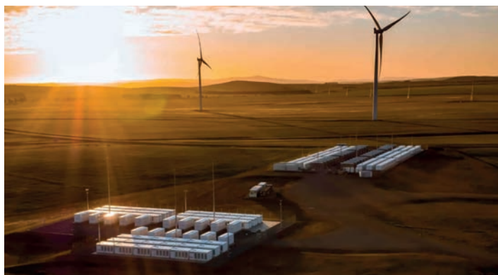
Hornsdale Power Reserve and Hornsdale Wind Farm
