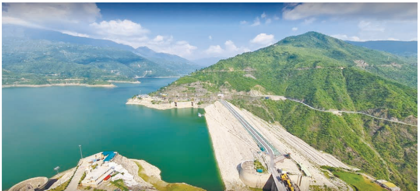
1,000 MW Tehri Pumped Storage Project, India
