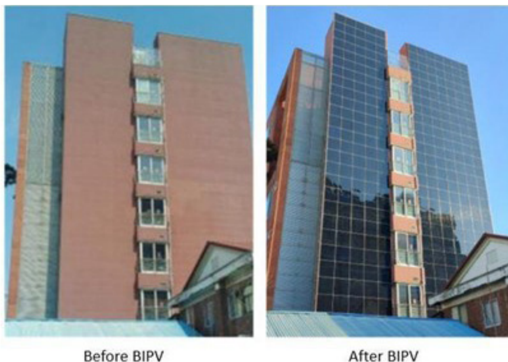
Figure 7: Before and after BIPV installation of Seoul SilverLight Hospital (translated and adopted from Energy Economy News, 2023)
